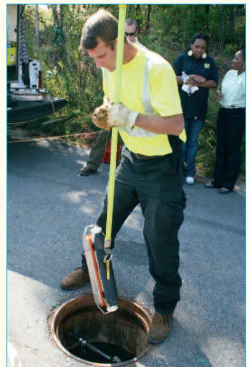
The data collected by the RedZone Solo Unmanned Inspection Robots has been analyzed and the results provide a list of rehab priorities.
