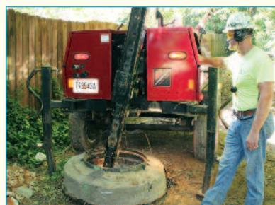
Jason Lovin, Foreman with RDJE, Inc., monitors the pipe bursting technology used to rehab nearly 3,000 linear feet of sewer lines within the Westpark area of the sewer system.
