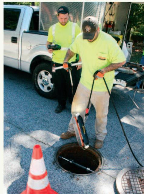
RedZone's Tony Frank lowers a Solo Unmanned Inspection Robot into a manhole to begin inspection and data collection of the condition of PCWASA sewer lines.
