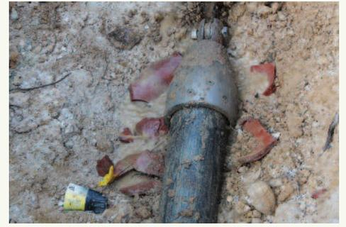
The pipe bursting method of sewer line rehab replaces aging vitrified clay pipe (in pieces around the new pipe being pulled) to improve the PCWASA collection system in areas that were previously deteriorating due to age.
