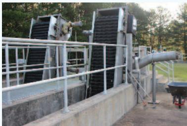
These two bar screens at the Rockaway Water Reclamation Facility are being replaced with newer, more efficient models to improve the wastewater treatment process at the plant.
