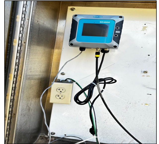
New turbidity meter install
