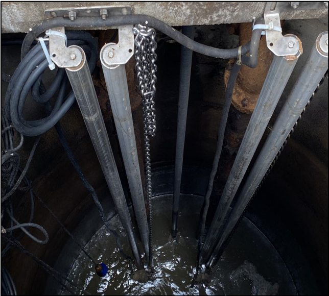
New rails at lift station
