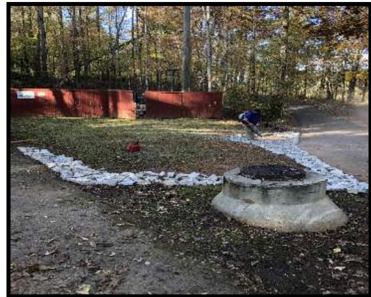
Erosion Control at Lift Station 27
