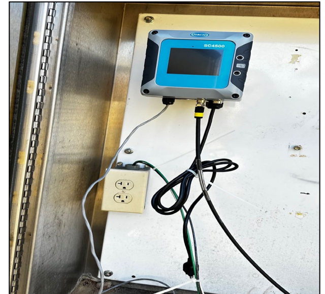
New turbidity meter install
