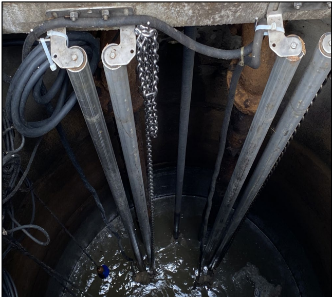
New rails at lift station
